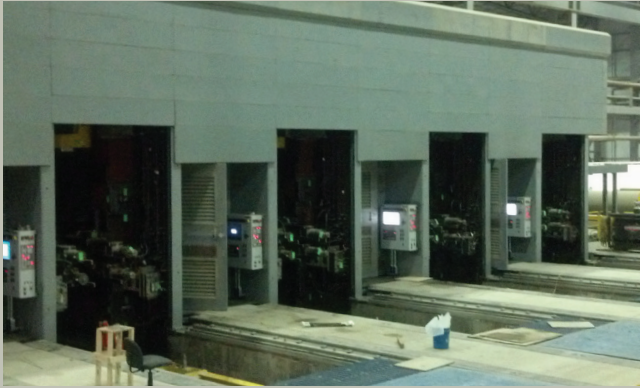
Mill stands dressed out and ready for commissioning
