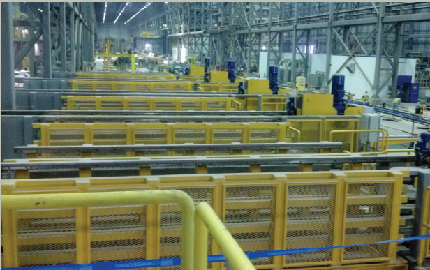
Automatic roll change cars to get the work rolls that will be put into the mill stand
